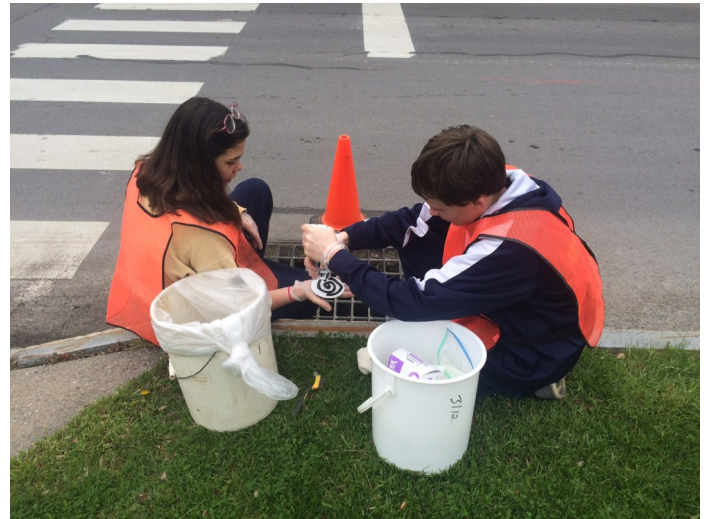
Storm drain marking!
