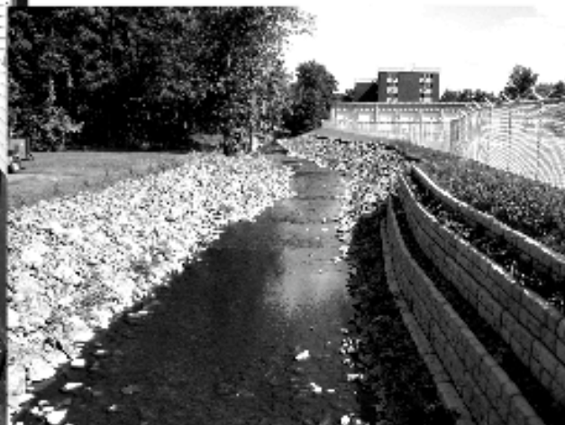
Completed project looking south from RG&E footbridge
