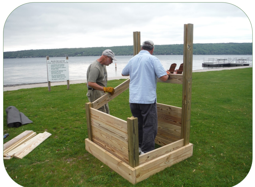
Volunteers installing a disposal station on-site at Onanda Park
